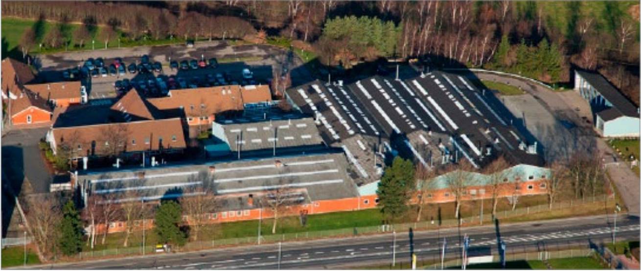
10,450 m 2 factory in Denmark, Headquarters of: scansteel foodtech A/S & Koncept Tech ApS
